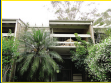
Close proximity to Nelson Bay CBD and treed outlook saw this townhouse sell in the high $200's
